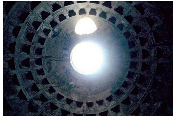
Figure 3: Perspective distortion in the detailed coffering geometry at the Pantheon, Rome (photo by permission Robin Benson, ©2003 R. Benson)
